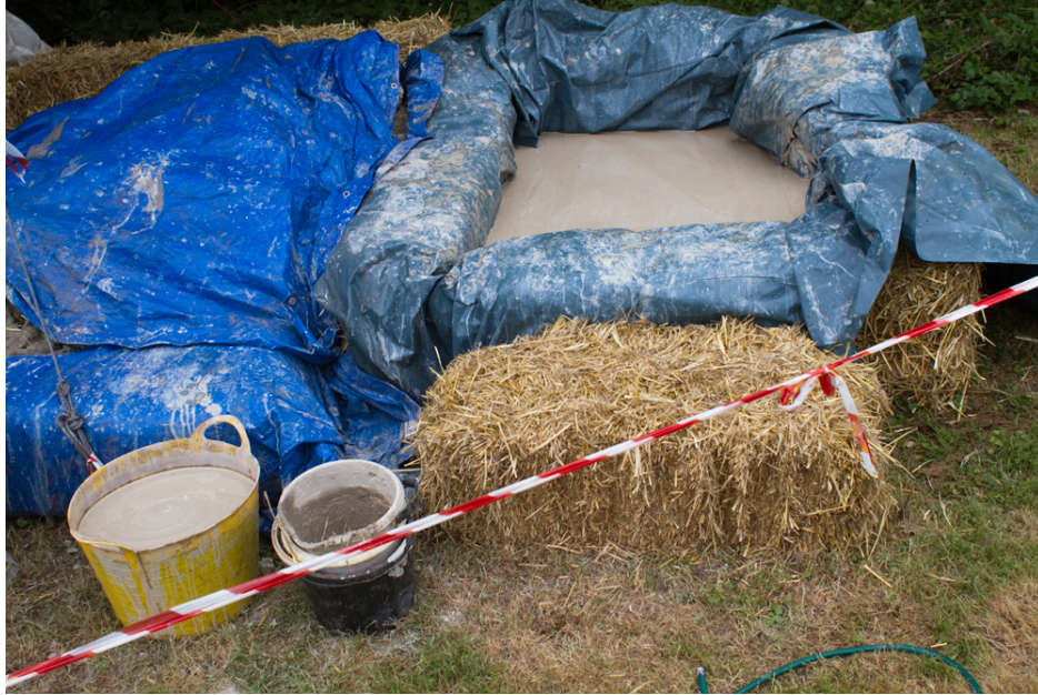
Making the clay slurry to mix with two parts sharp sand and one part straw for the cob mix
