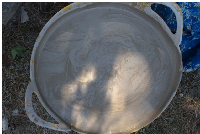
After a 48hr soak the clay slurry is ready for the 'key' layer
