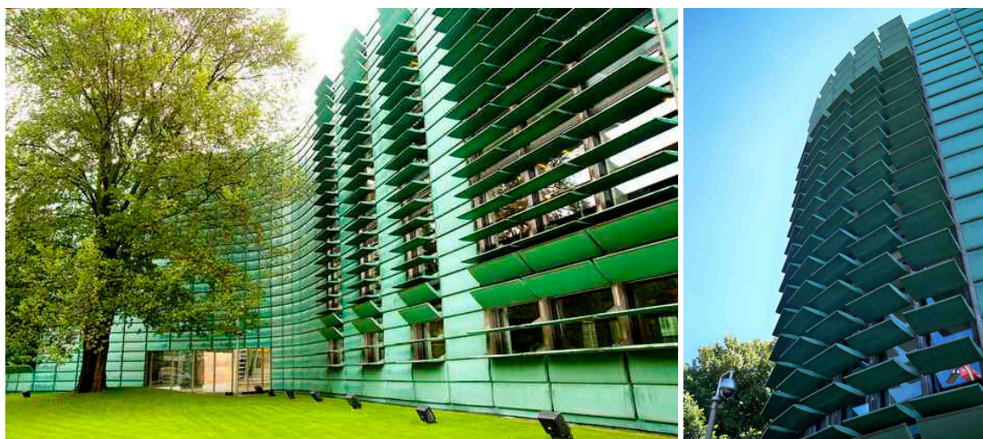
Figures 10 & 11. Pan- Nordic Embassy, Berlin (various architects – completed 1999). Six architectural firms collaborated, with one firm taking charge of the master plan and unifying ‘skin’, a ribbon of operable copper louvres that surround the complex, bringing cohesion to the design. This is a fine example of successful design collaboration.
