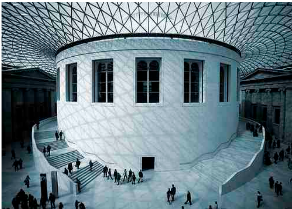
Figure 5. New Dome over the Great Court at British Museum, London (Foster, 2000) Complex form buildings such as these such as these are not possible without today's computer-assisted design technology
