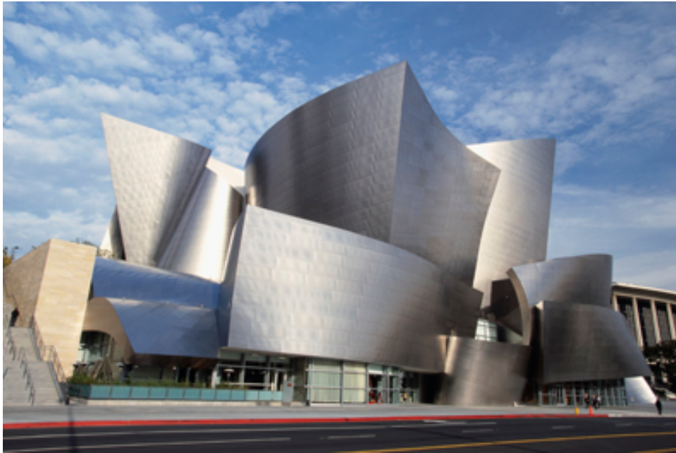
Figure 4. Walt Disney Concert Hall, Los Angeles (Gehry, 2003)
