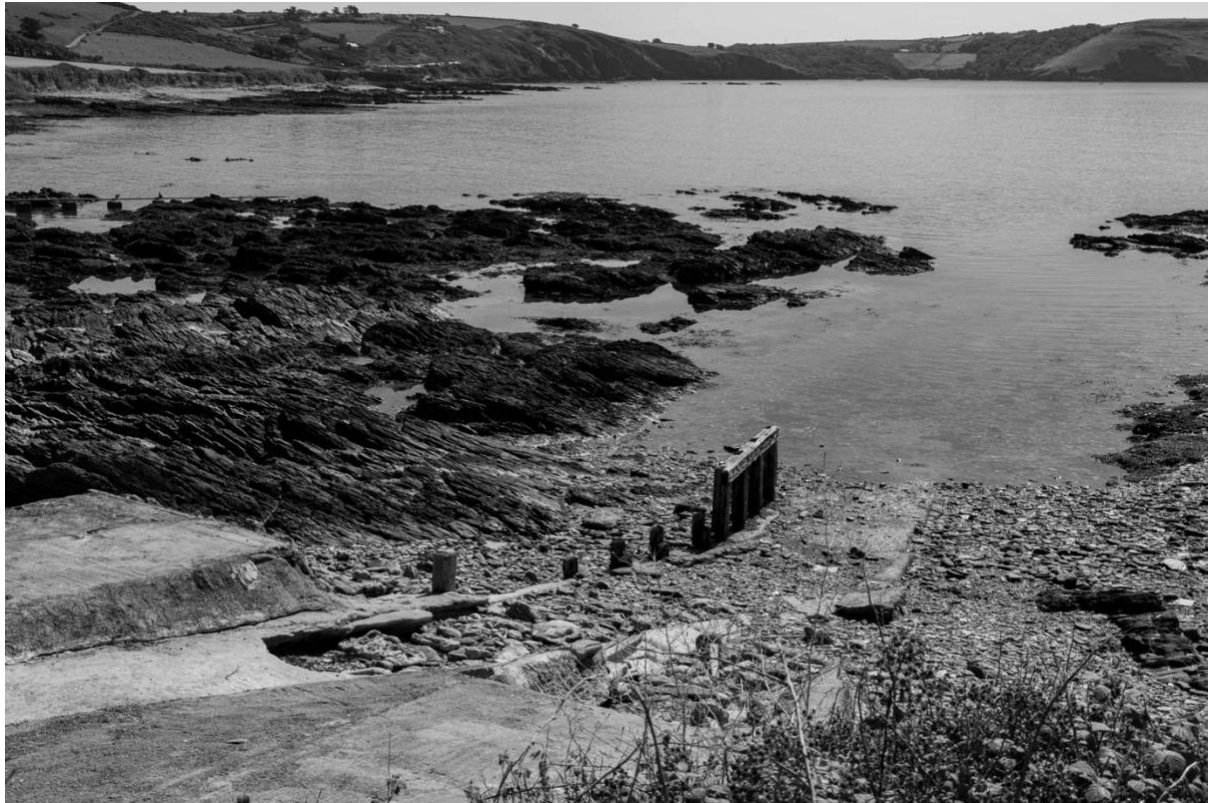
Remains of a concrete ramp and wooden pier (Photo: L Hodsdon)
