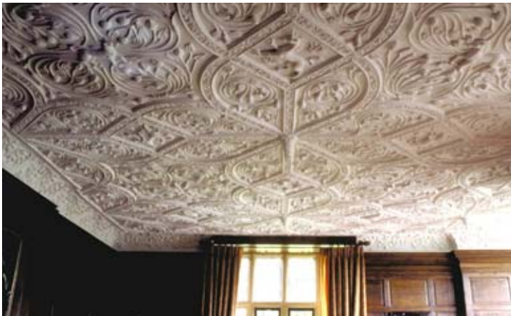
Fig. 5 One-off strapwork ceiling produced by Hayles & Howe
