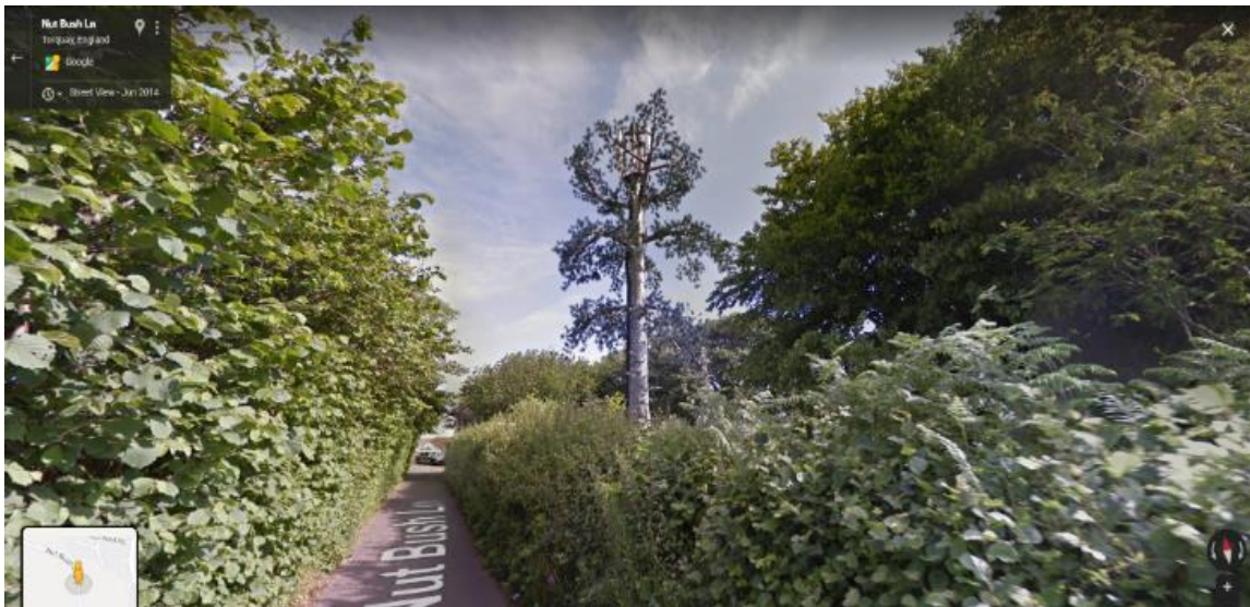
Fig. 57- Cell mast disguised as tree. Google Street View.
